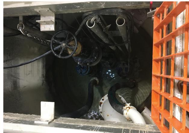
GPM-Eliminator Submersible Pumps in Water Treatment Process
